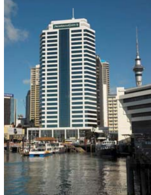
Pricewaterhouse Coopers Tower
