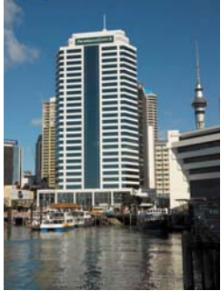
Pricewaterhouse Coopers Tower
