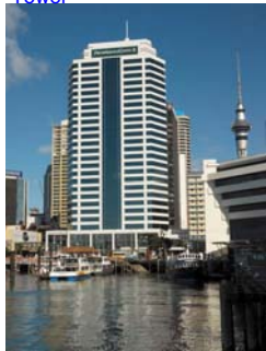
Pricewaterhouse Coopers Tower
