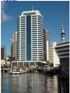
Pricewaterhouse Coopers Tower
